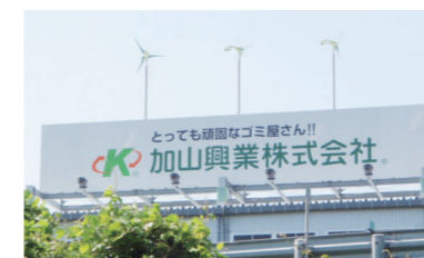
Wind power generation system
